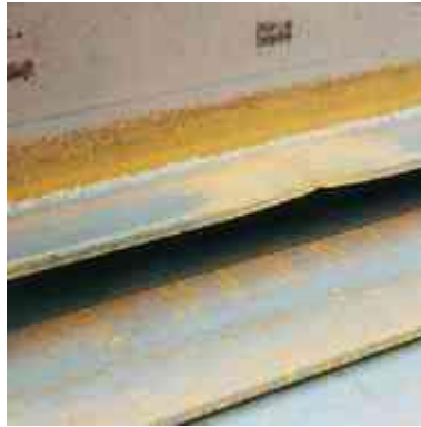
No. 24 Large steel beams
