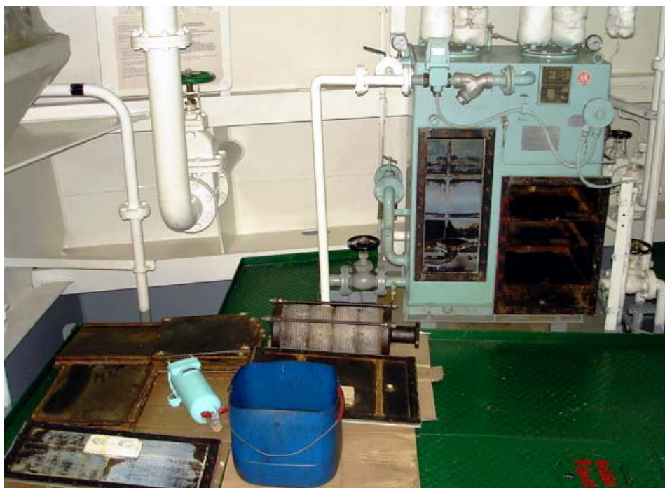
OWS opened for maintenance
